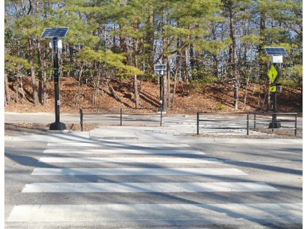
An at-grade greenway crossing on Maynard Road
