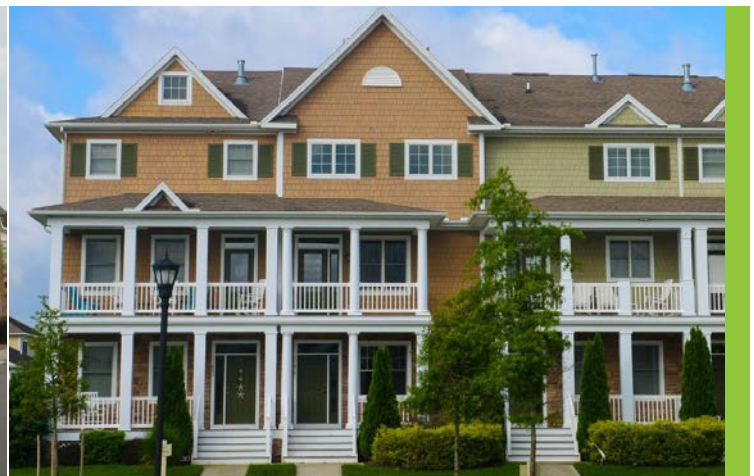
Attached single family and multifamily housing
