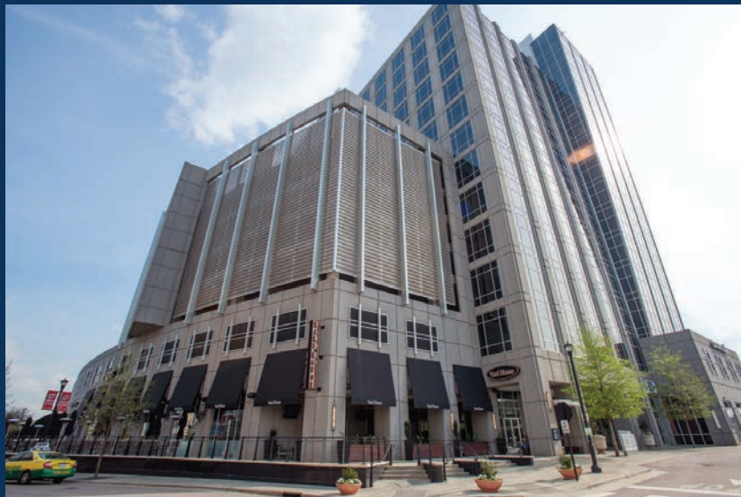
Taller office buildings are a key part of the mixed use development of North Hills in Raleigh.
