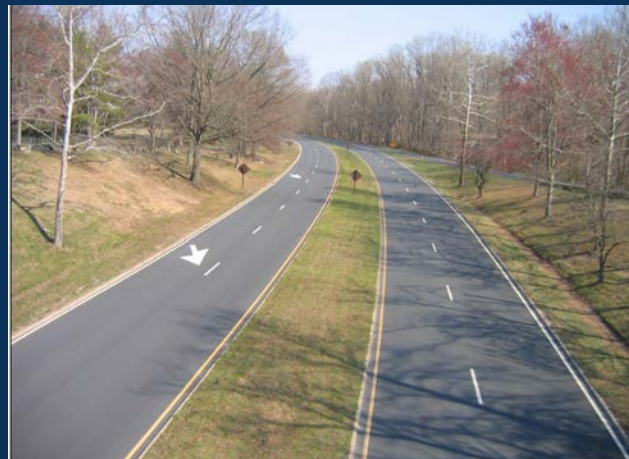
The rural thoroughfare pictured to the left has a very simple median, planted with grass. This sort of median landscaping is more appropriate for historic contexts. Note also the use of a very simple curb to stabilize the outer edge of the pavement.
